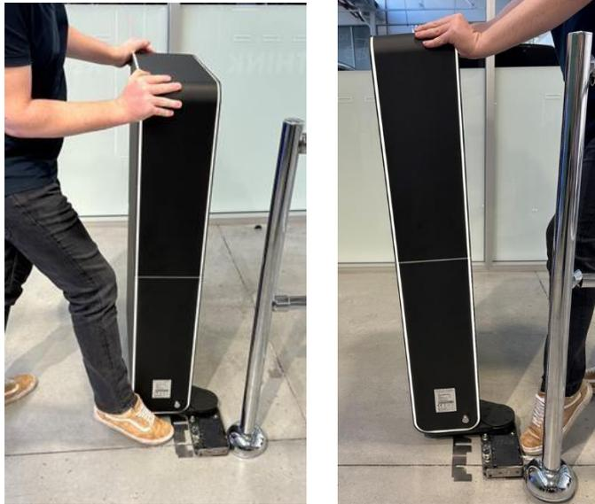
Check for floor clearance now that the gate has been lifted and assess if a larger plates are required.
