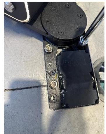
Tilt the gate to one direction and slide one half of the bracket underneath. Then tilt the gate the other direction and slide in the other half of the bracket underneath the gate. (See image below)
